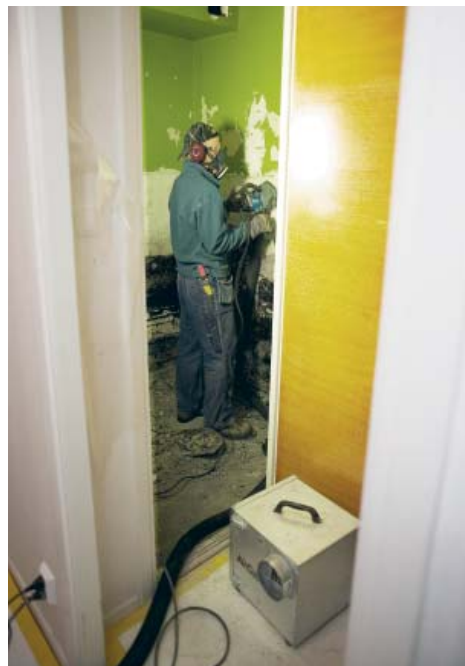
By circulating the air through a highly efficient HEPA filter, the air in the room is cleaned from airborne dust.
